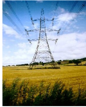
Figure 2: 240kV Transmission tower
