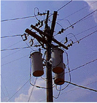
Figure 1: 25kV Distribution pole – deadend structure with transformers
